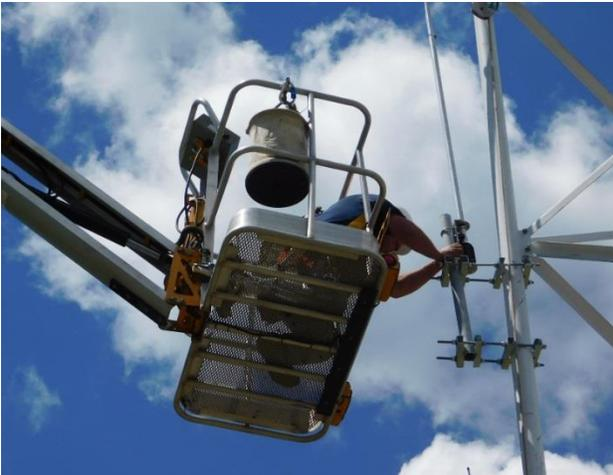
*Mounting the Comet HF antenna.*
